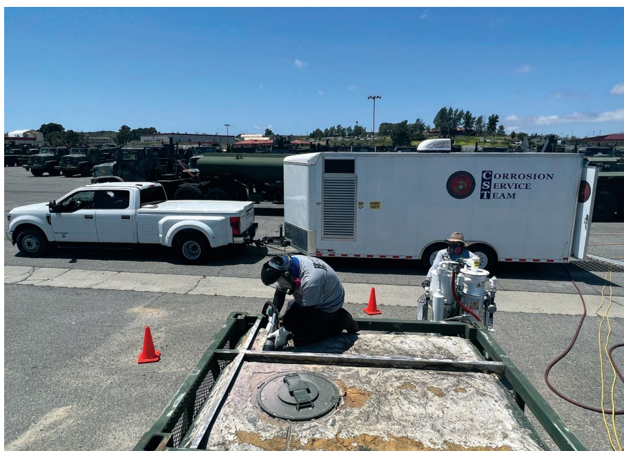
A CST technician employs a mobile blast recovery system—an example of the enhanced capabilities researched and utilized by the CPAC Team—to perform condition-based corrosion repairs. (CPAC Team Files.)
