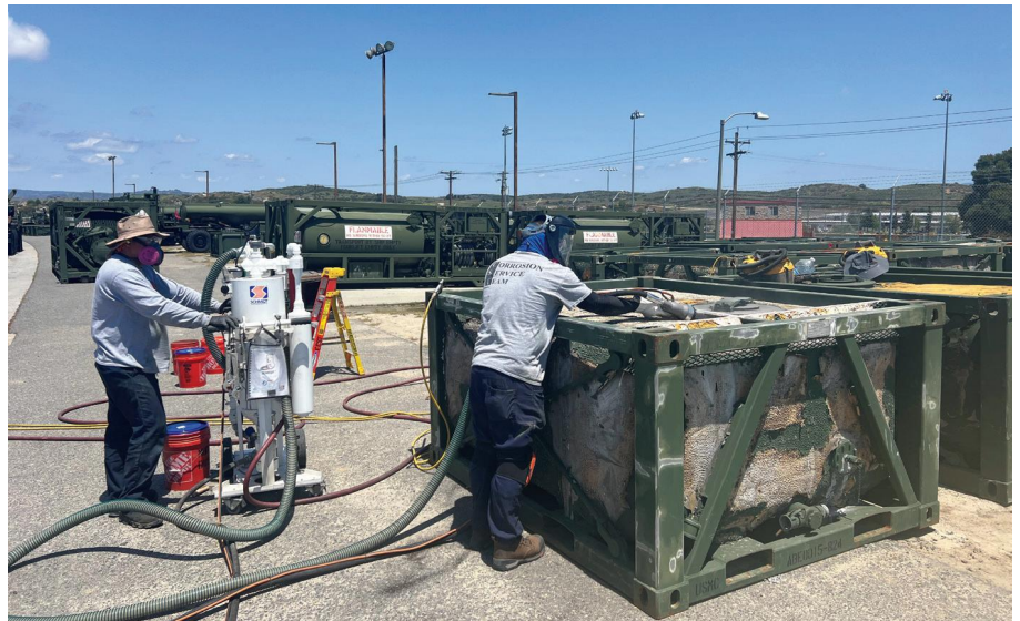
Corrosion Service Team technicians perform enhanced surface preparation and touch repairs on a water sixcon container at a supported unit's location. The CPAC Program employs intermediate-level corrosion repairs using enhanced capabilities. (CPAC Team Files.)
